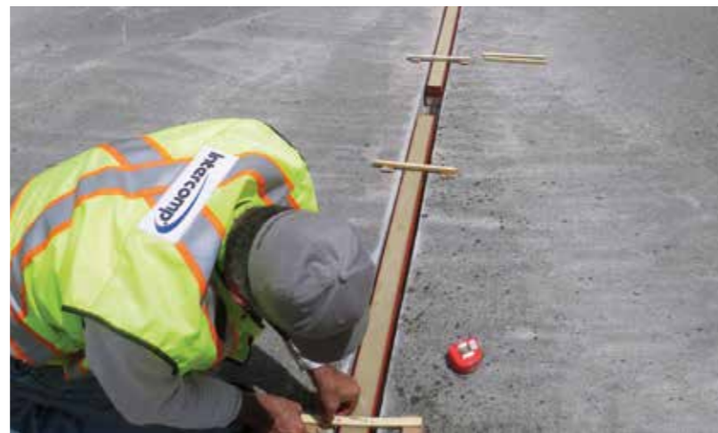
(Above) Intercomp's strain gauge strip sensor (Right) Accurate data collection from the WIM system (Below) Installation can be completed within eight hours
