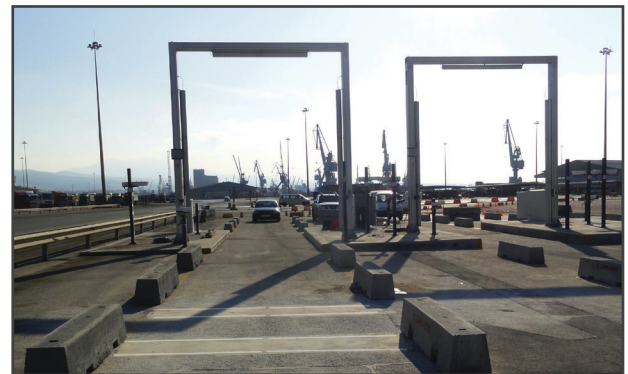
In-ground installation of port dynamic weighbridges in Thessoloniki, Greece
