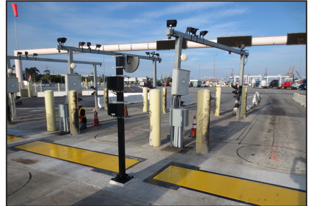
Low-Speed Weigh-In-Motion (LS-WIM) scales automate gate processes saving time and man hours.
