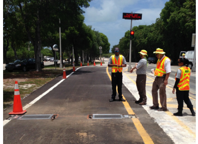
The LS630 scales were inset within the lane at the weighing site
