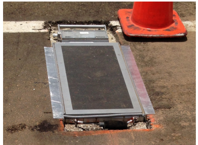
Saw cuts made within pavement for scale placement.
