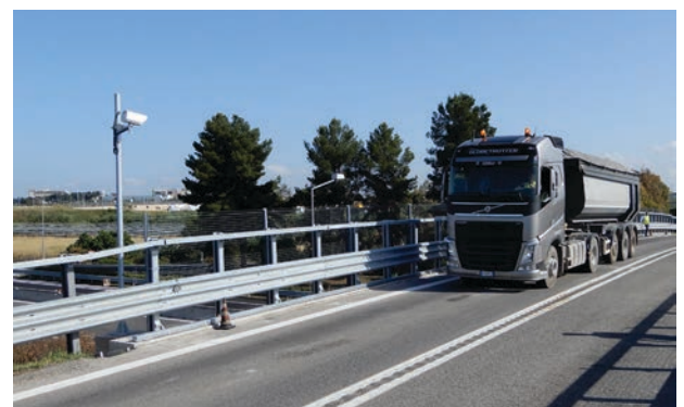
WIM sites identify overweight trucks to minimize impact on roadways and bridges.
