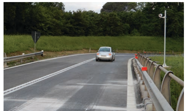
Sensors are ground flush with roadway surface and are combined with ANPR cameras for vehicle identification.
