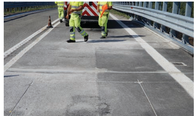
Strip Sensors are installed in the traffic lanes to weigh vehicles without stopping.
