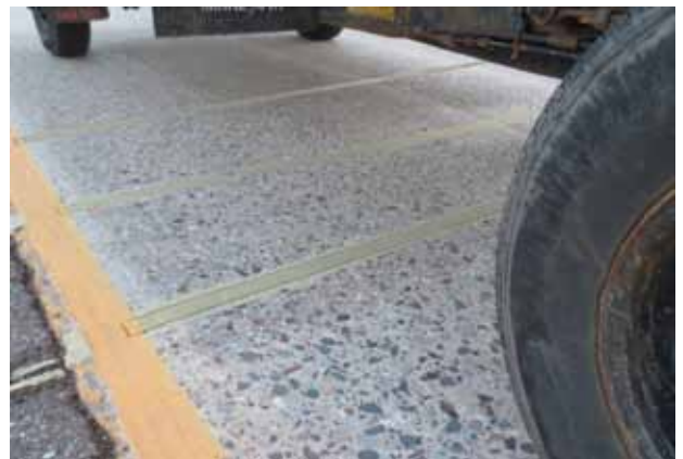
Strip Sensors can be installed in a single day for WIM operation across a wide speed range.
