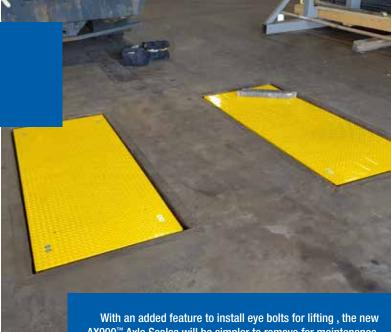
AX900<sup>™</sup> Axle Scales will be simpler to remove for maintenance.
