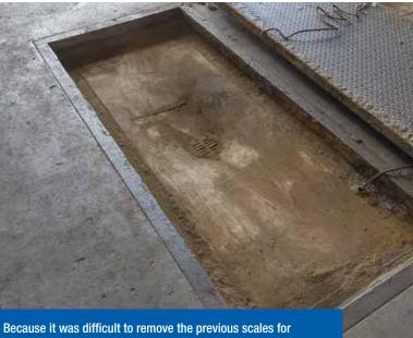
maintenance, moisture and dirt accumulated within the pit, ultimately leading to the scales failing.
