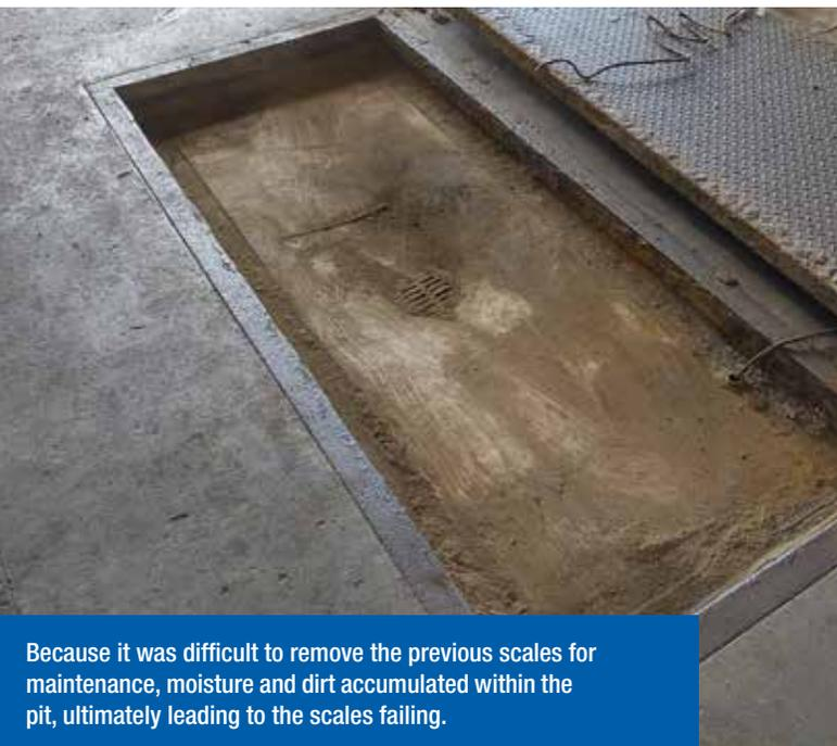
Because it was difficult to remove the previous scales for maintenance, moisture and dirt accumulated within the pit, ultimately leading to the scales failing.
