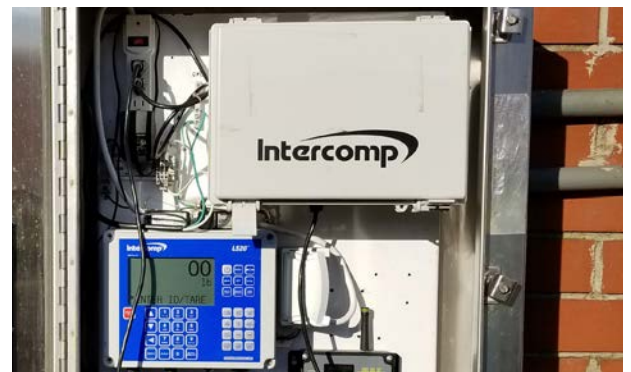
The LS20 ™ WIM Indicator computes and stores weight data for later usage. The weather resistant printer allows plant managers and truck drivers to print physical weigh tickets.
