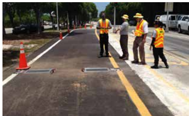
The LS630-WIM™ scales were inset within the lane at the weighing site.
