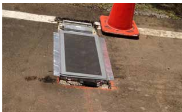
Saw cuts made within pavement for scale placement.
