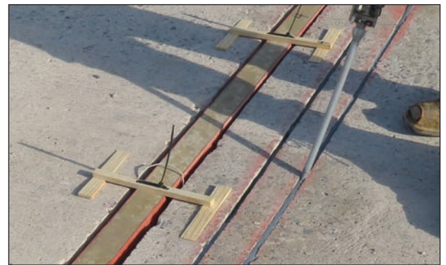
Sensors are placed in channels cut in pavement, with no drains required, and grouted in place.
