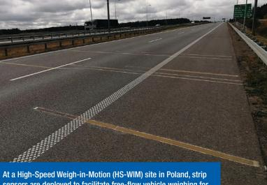
At a High-Speed Weigh-in-Motion (HS-WIM) site in Poland, strip sensors are deployed to facilitate free-flow vehicle weighing for all traffic, including vehicles traveling on the highway shoulder.
