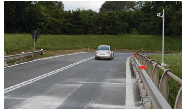
Sensors are ground flush with roadway surface and are combined with ANPR cameras for vehicle identification.
