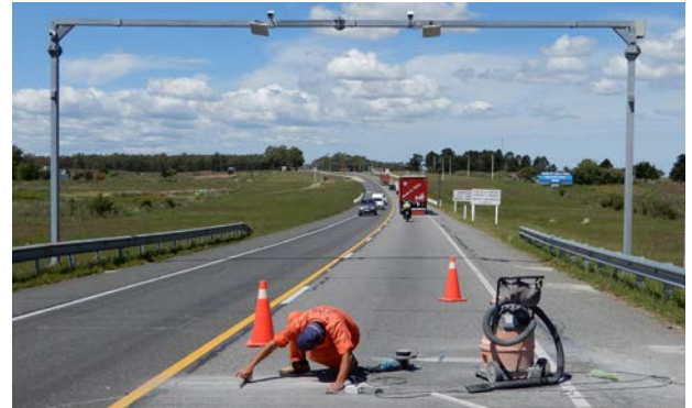
Intercomp Strip Sensors in the highway upstream of the weigh station.
