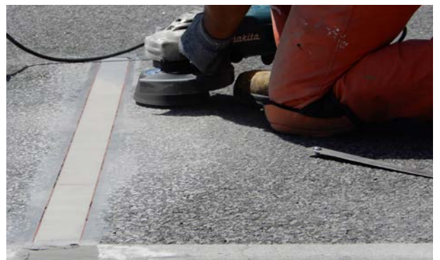
Sensors are installed in the pavement and ground flush with the roadway surface.
