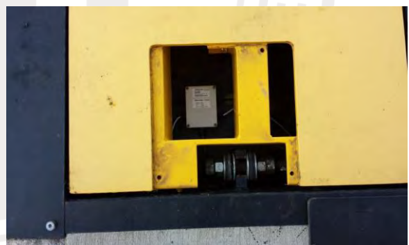
Access Cover removed showing junction box and data badge
