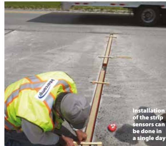
WIM site screening for enforcement in the USA
