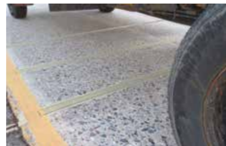
(Above) Three pair configuration of sensors installed in concrete
