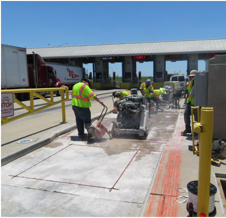
Installation is simplified with a loop sensor and flush-mounting the strip sensors into shallow cuts, reducing costs and operational disruptions.
