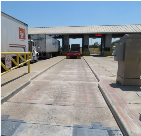
Installation is simplified with a loop sensor and flush-mounting the strip sensors into shallow cuts, reducing costs and operational disruptions.
