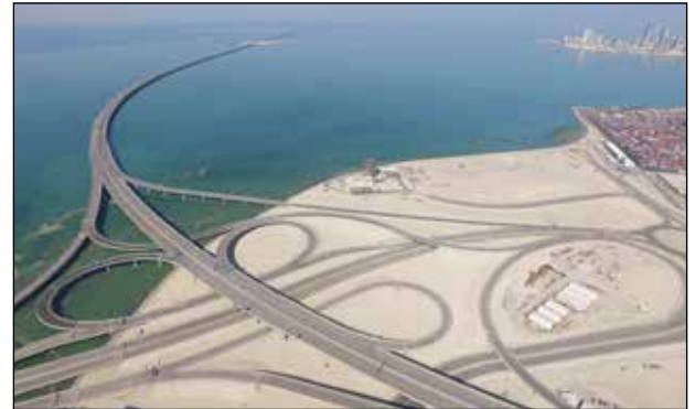
Kuwait's new causeway represents a large investment in infrastructure, with the requirement for protection from overweight vehicles.
