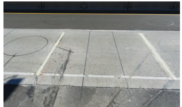
Mainline pre-screening WIM strip sensor installations have 4 sensors in a dual-threshold configuration.
