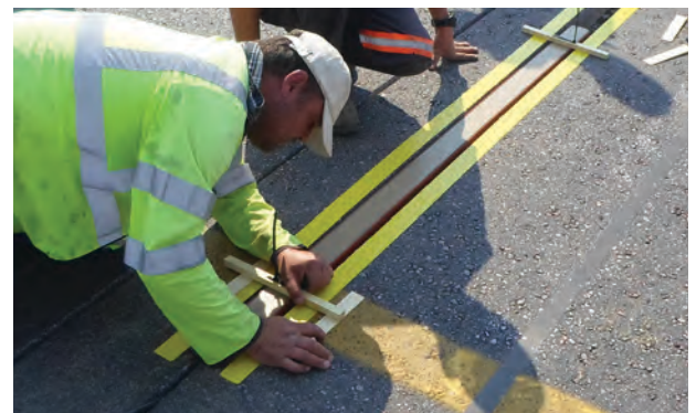
Intercomp sensors are embedded in 3" (75 mm) channels cut into the pavement.
