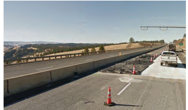
When resurfacing the mainline, ODOT removed frame-based scales and replaced with WIM Strip Sensors.
