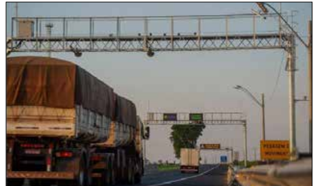
As a result of the weights and vehicle dimensioning, vehicles can be directed by VMS to exit for further actions.
