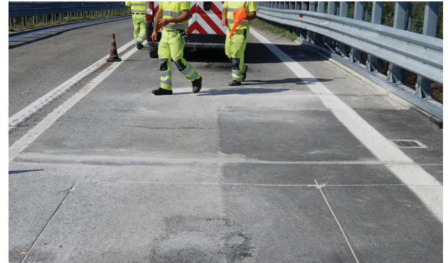
Strip Sensors are installed in the traffic lanes to weigh vehicles without stopping.
