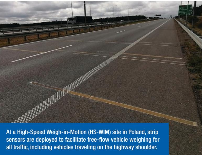
At a High-Speed Weigh-in-Motion (HS-WIM) site in Poland, strip sensors are deployed to facilitate free-flow vehicle weighing for all traffic, including vehicles traveling on the highway shoulder.
