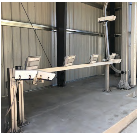
REMPRESX AGS automated freight checkpoints are replacing conventional manned gates at the intermodal terminal.
