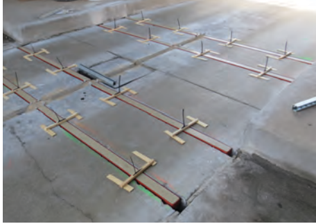
Pairs of Intercomp's WIM sensors were easily and quickly installed with little disruption to the terminal's operations
