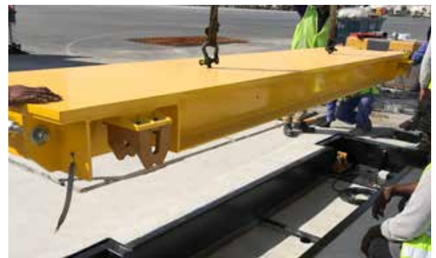
The small footprint of these scales allows them to be installed in a matter of days, keeping downtime to a minimum.
